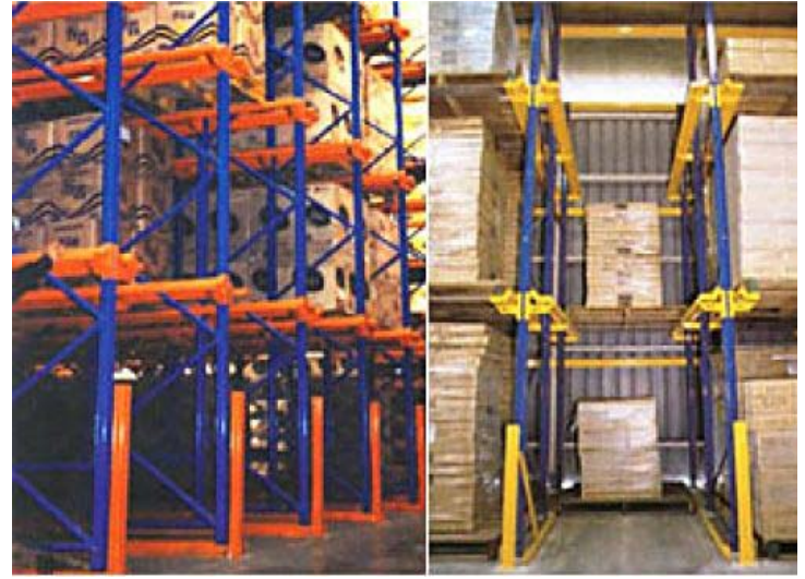
Drive in Drive Through Racking
